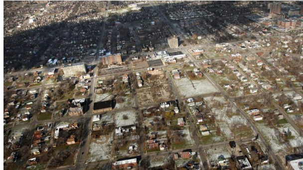
Figure 7: Detroit Public Relations: Image showing state of disrepair, Detroit 2009
